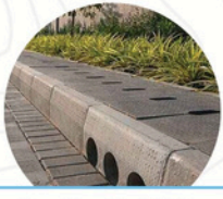
Footpath With Curbing Stone
