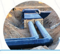
Under Ground Drainage
