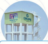
Over Head Tank
